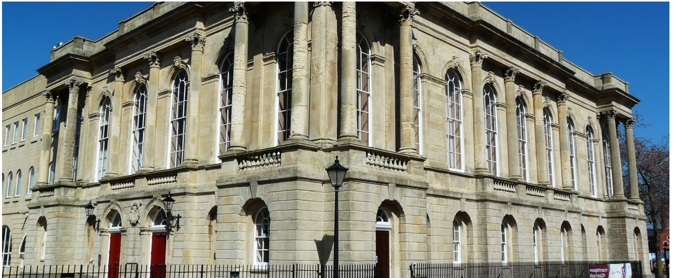
The Dylan Thomas Building of the University of Wales incorporates an entrepreneurship hub, event space and cafe
